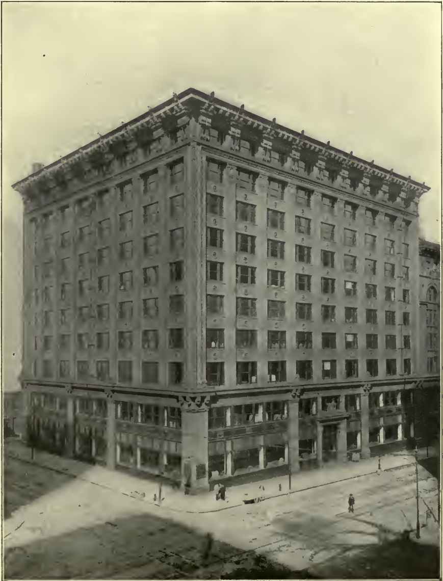
BUILDING OF THE CARLETON DRY-GOODS CO. St. Louis, Mo.
